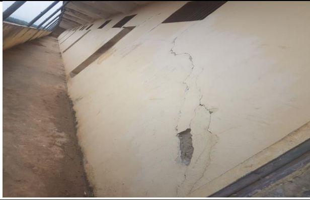
Block 1 of Mafanta detention facility before refurbishment (visible cracks, no painting, no grills along corridor)
