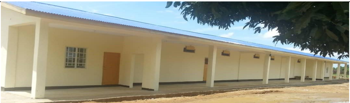
Progress on the refurbishment of the Waterloo Correctional Facility. Up: dilapidated building at the start of the refurbishment work. Down: refurbished building to host at least 150 inmates, contributing to decongest already overcrowded facilities
